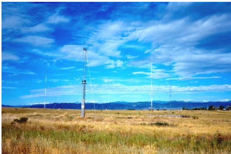
(FIGURE 1) This is a picture of the 15 MHz antenna from WWV. The 10 MHz are of a similar design. Source: National Institute of Standards and Technology (NIST) ( http://file:///C:/Users/HP/AppData/Local/Packages/microsoft.windowscommunicationsapps_8wekyb3d8bbwe/LocalState/Files/S0/3/Attachments/sp250-67[4043].pdf ).
