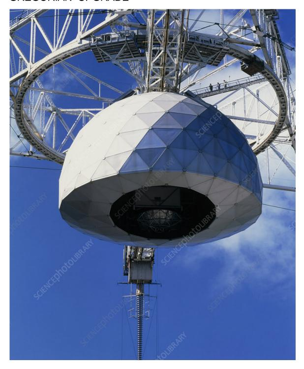
A second upgrade was carried out in the 1990s when Per-Simon Kildal and others designed a Gregorian dual reflector system that was enclosed in an 86 foot diameter protective dome. This allowed a rotating floor of different point feed horns to be moved into a single focus thus correcting the spherical aberration and not being limited by the narrow bandwidth of line feeds.
