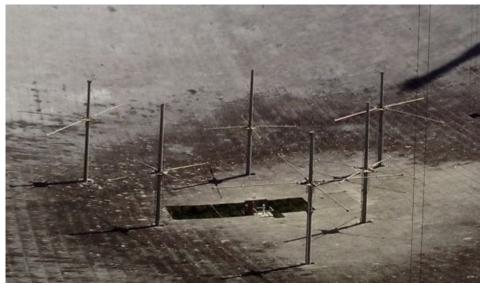
In 1998, the HF heating (ionospheric modification) facility located about 10 km along the coast was destroyed by Hurricane Georges. This facility had a design that consisted of 32 pyramidal log periodic antennas covering 3 to 12 MHz and a power of 600 kW. It was used to modify the ionosphere effectively creating a plasma research laboratory in the sky. The 430 MHz ISR was then used as a diagnostic tool to measure the effects of the ionospheric heating.
