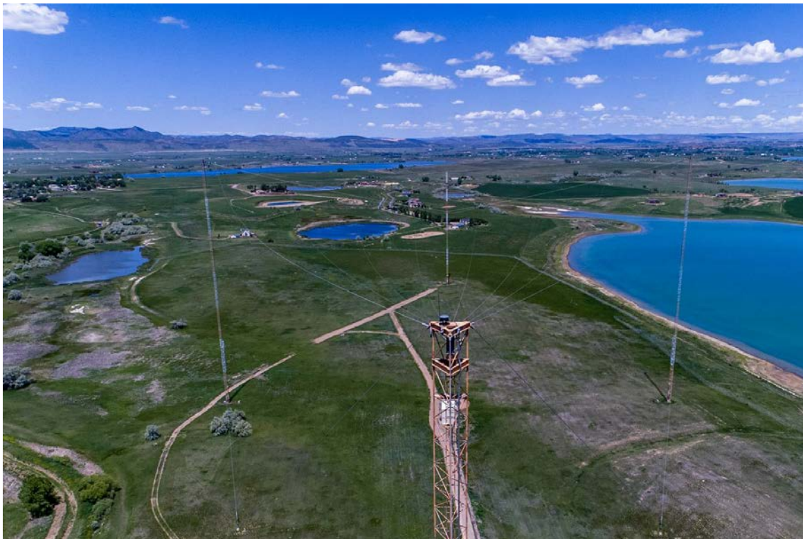
WWVB North Array towers and capacitive "top hat" network of wires. Aerial drone photography by Dave Winnett, WØDDZ
