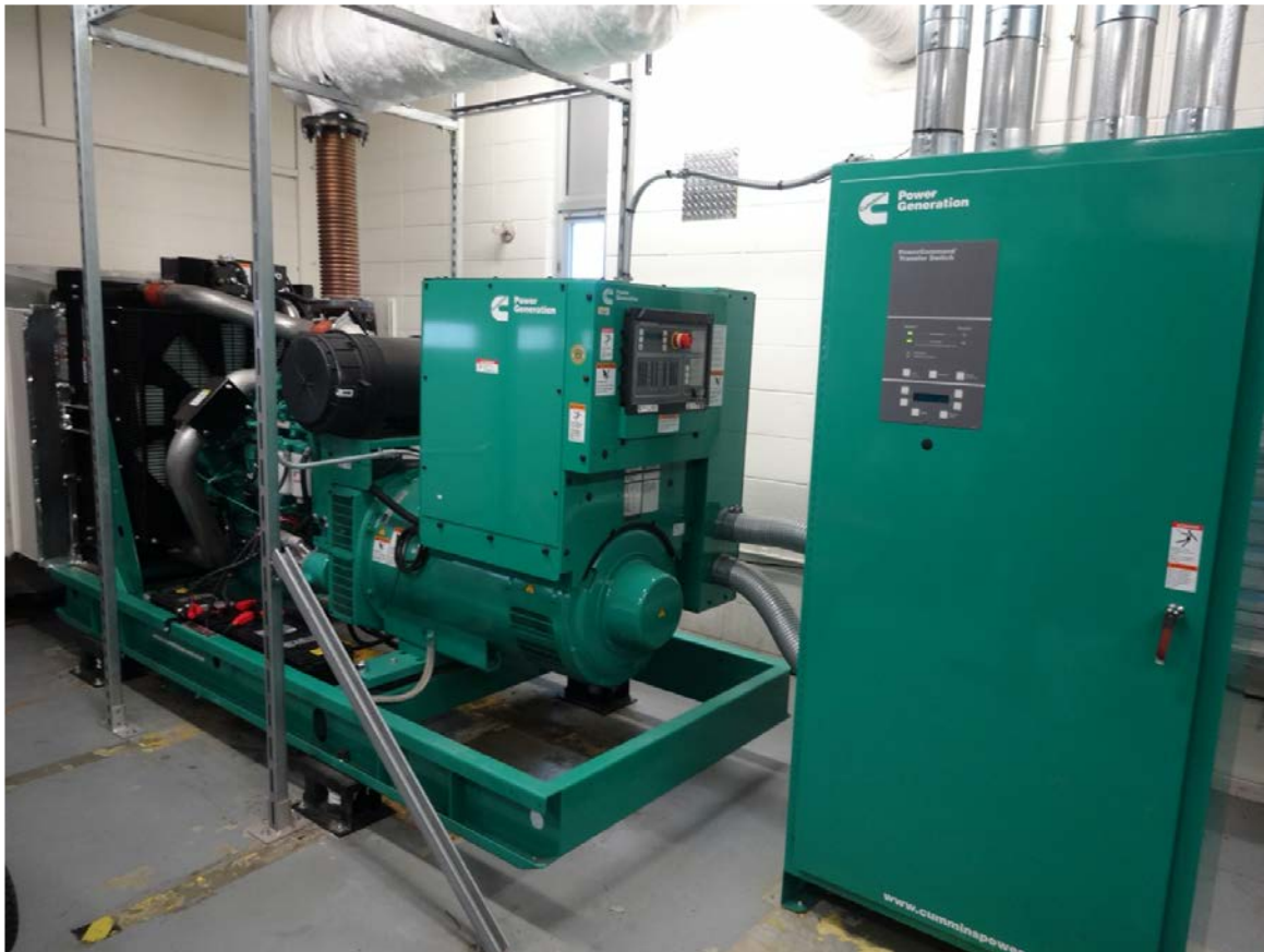
WWV 250 kW back-up generator. photo by Fred Schwierske, W9KEY
