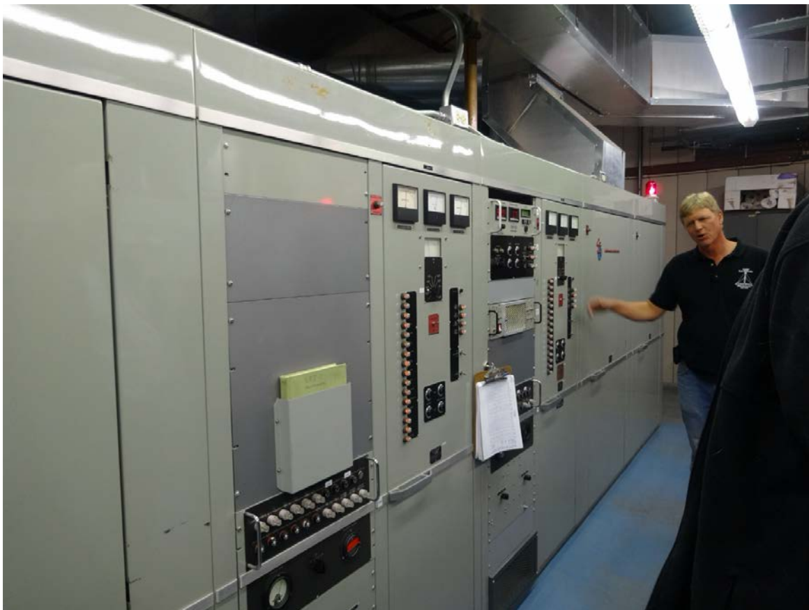
NIST station employee Bill Yates, KE0UZZ, explains the operations of one of WWVB's three Continental Electronics 50 kW transmitters.
