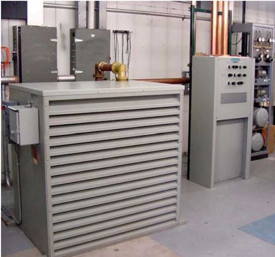
The WWVB dummy load (left) and the Matrix Switch (right) which is being replaced with an automated switch. photo by Fred Schwierske, W9KEY
