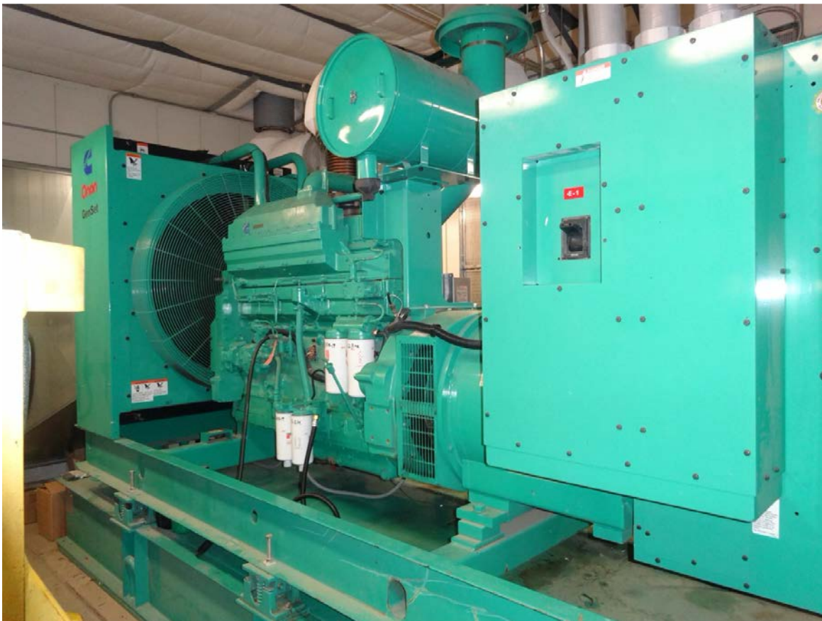
WWVB 500 kW back-up generator. photo by Fred Schwierske, W9KEY
